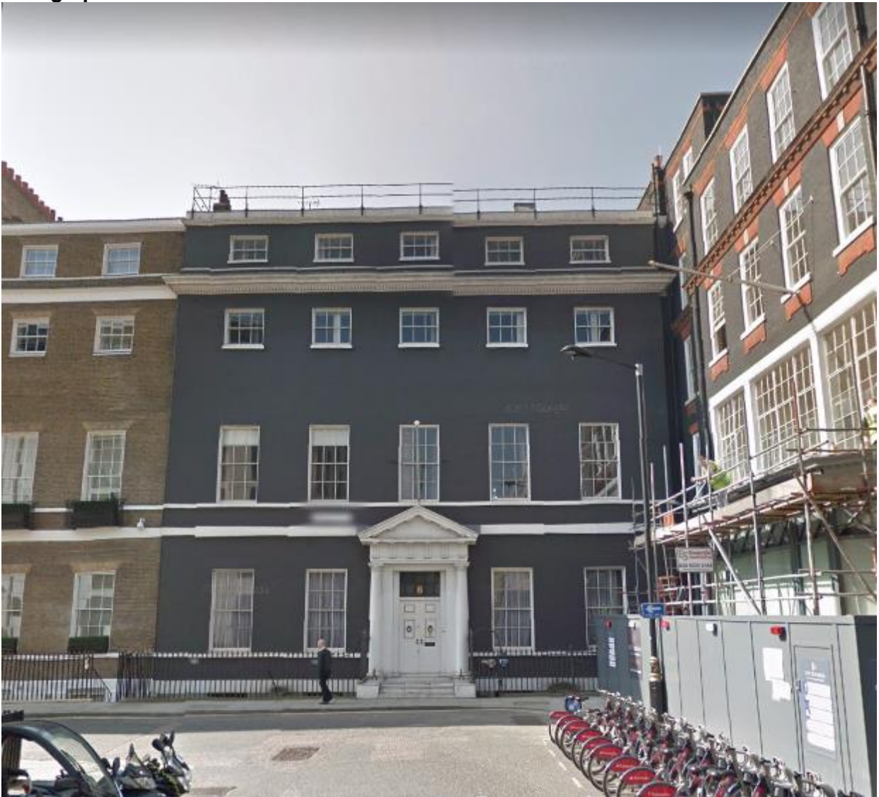
Photograph 1: Grafton Street elevation
